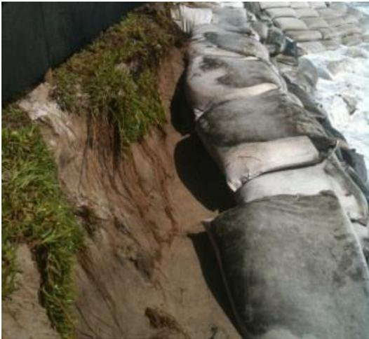
**6. Erosion of crest backfill (from overtopping)**
